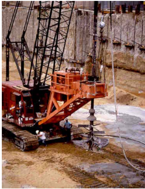
Figure 1. Shallow Soil Mixing Equipment
